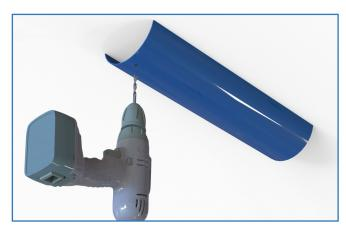
2. 30mm in from either edge of the jointer, using the 6.5mm drill bit, drill a hole through the jointer and gutter. Remove the jointer and debur the holes if necessary.
