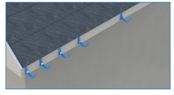
2. Secure first gutter bracket with 5mm x 50mm stainless steel screws. Fix one screw and set to a string line as required.
