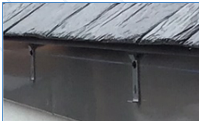
Fig 2. Bracket in place at 500mm centre-to-centre.
