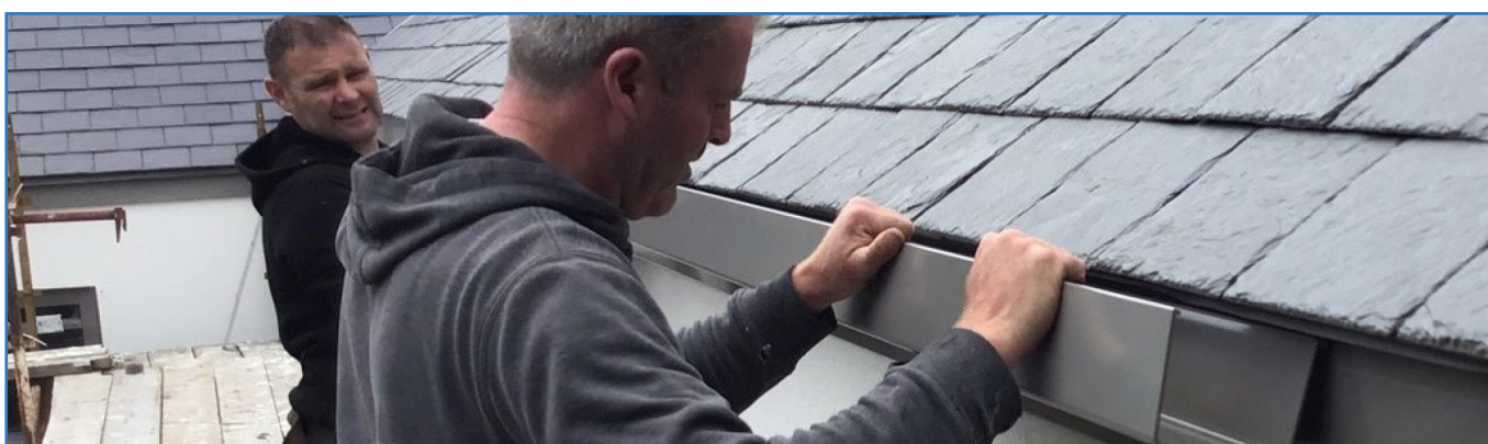
Fig 3. Gutter hooked on top of fascia bracket prior to being snapped in place.
