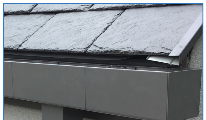
Fig 5. Outlet and End cap in place.
