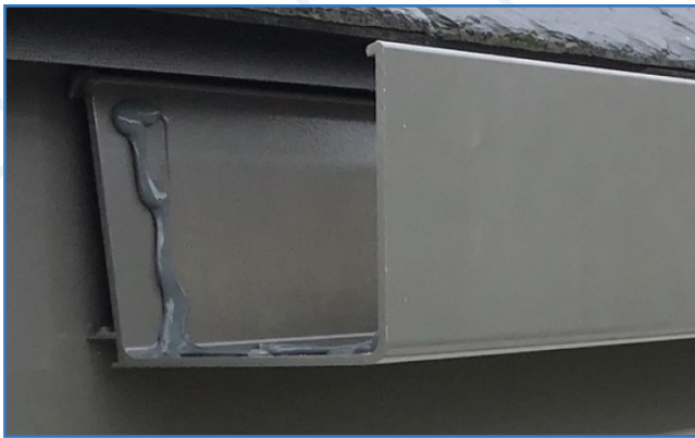
Fig 4. Fitted length with the high performance, low modulus sealant. bead in place.
